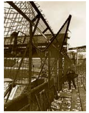
10ft high perimeter fence cut open to let fans escape
